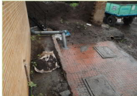
Oversized septic tanks
