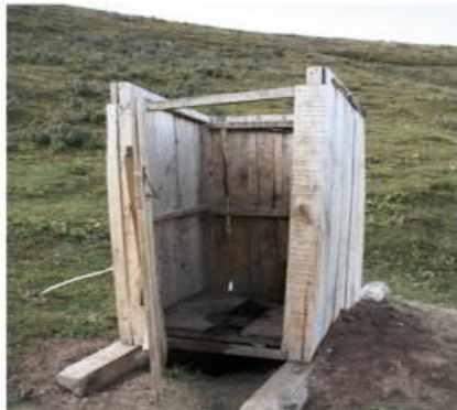
Single pit toilets
