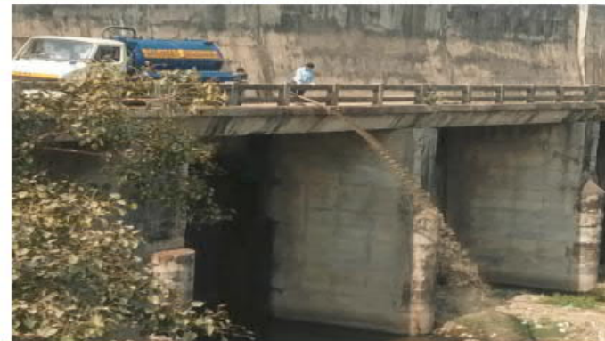
Disposal of septage in water bodies
