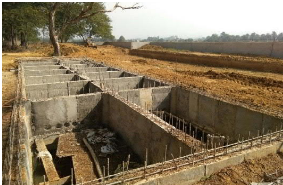
Anaerobic baffle reactor
