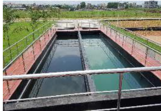
Settling cum thickening tank
