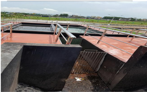
Inlet chamber and screen
