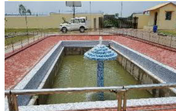
Polishing pond with aeration
