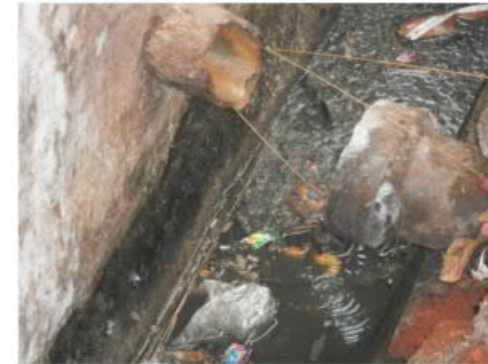
Toilets directly connected to drains
