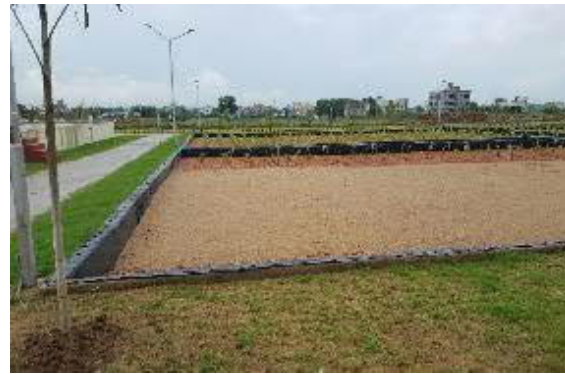
Planted gravel filters
