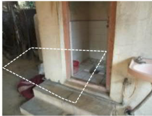
Inaccessible septic tanks with sealed tops
