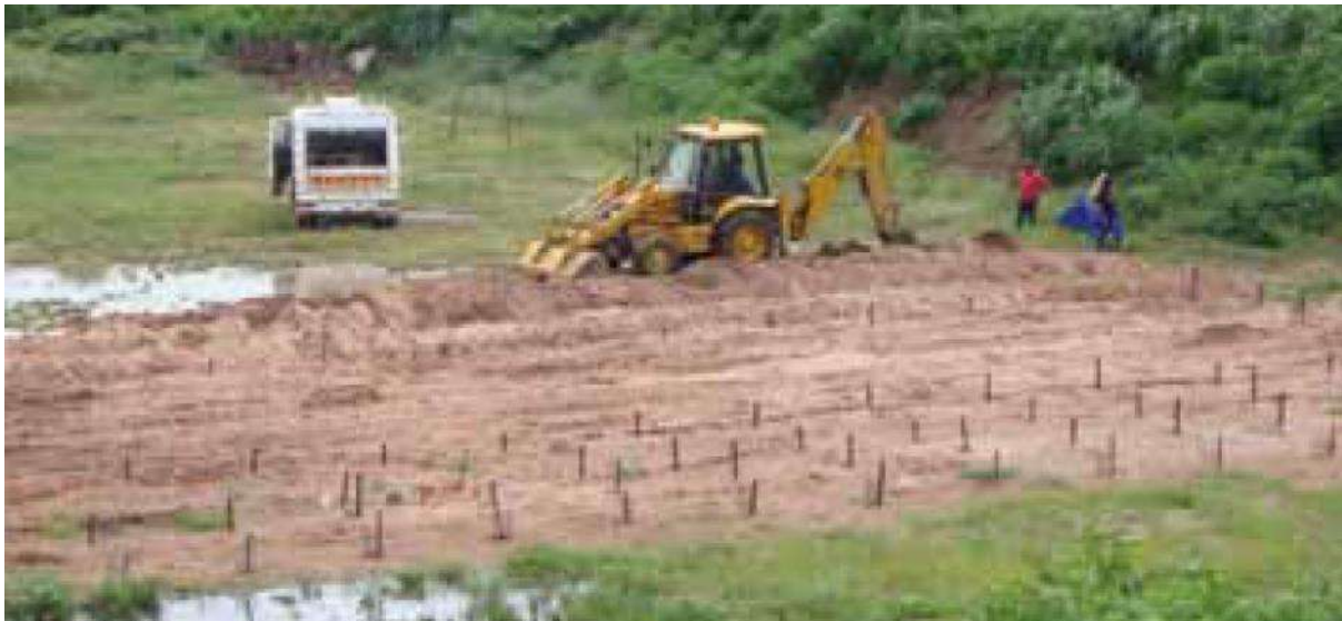
Figure 4-9: -Typical deep row entrenchment site
