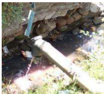
Figure 4-5 Toilet discharge directly into open drain
