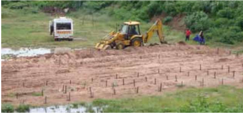
Figure 4-12 Typical deep row entrenchment site
