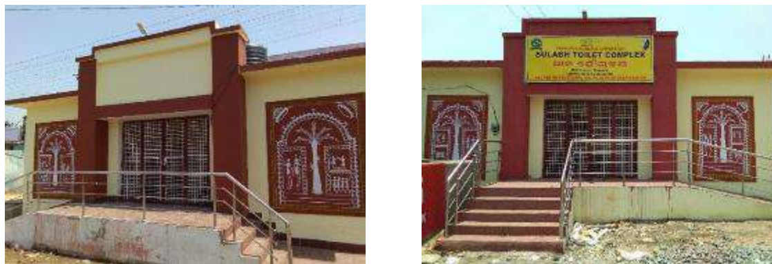
Figure 4-6 Five to ten seat - Newly constructed Hybrid unit at Burla bus stand and Bareipali
