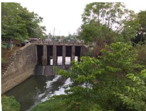
Figure 4-9: -Open drain in which faecal waste is disposed
